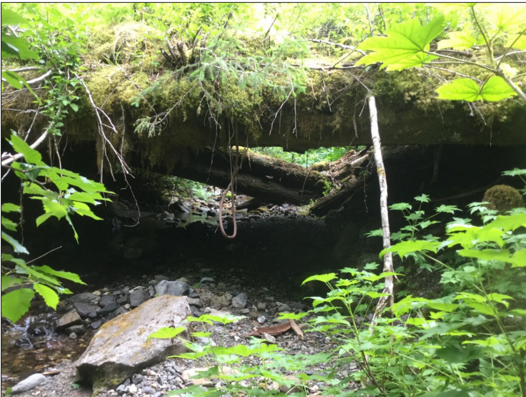
Figure 3.—Partially collapsed log-stringer bridge at waypoint 936.
